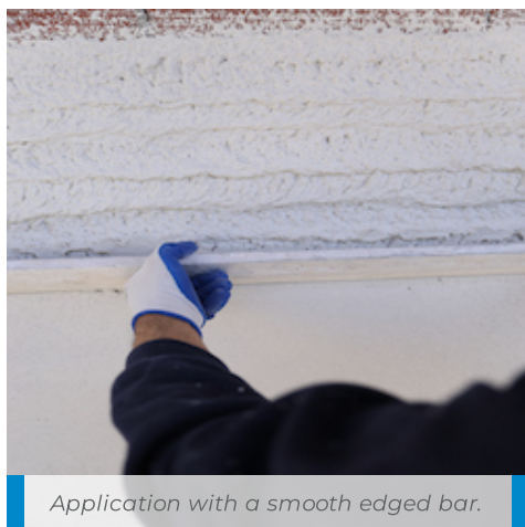
Finishing the surface of Intomap Mono.
