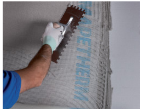
Application of reinforcing layer with Mapetherm Net
