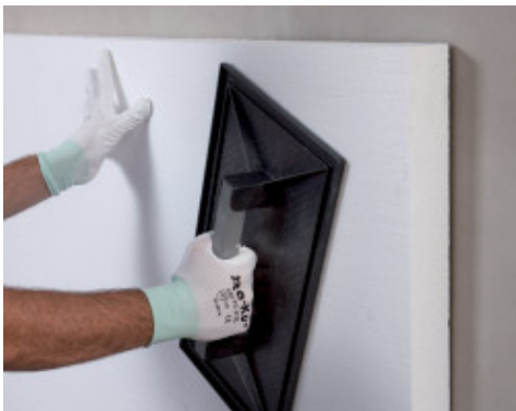
Apply pressure on the insulation panel to ensure good bonding with substrate
