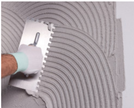
Application of first leveling layer of Mapetherm AR3 GG
